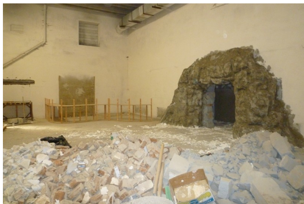
Stavba TEPfactoru Slapy. Construction of TEPfactor Slapy.
